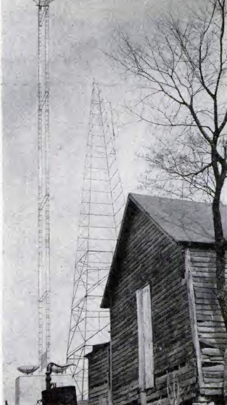
Above, microwave station near Pikes Peak, Ind., relays network shows to Bloomington from Cincinnati (see map below). Tower at left is used. Windmill tower at right was original installation. Transmitter is inside block house under "dishpans" at tower base
